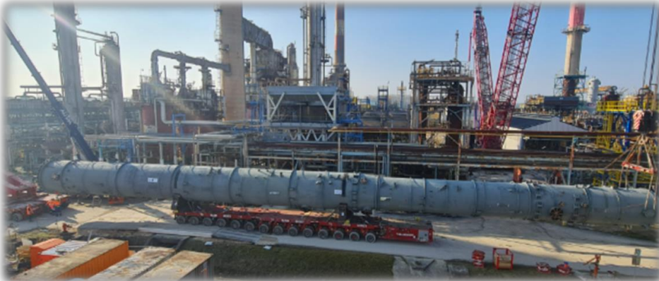
Fractionation column erection February 2025
